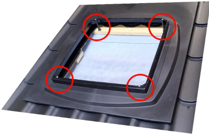
Picture 6. Fixing the base to the battens with screws through the support sleeves.
